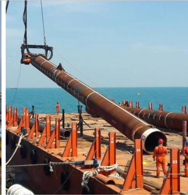
Driven pile anchor
