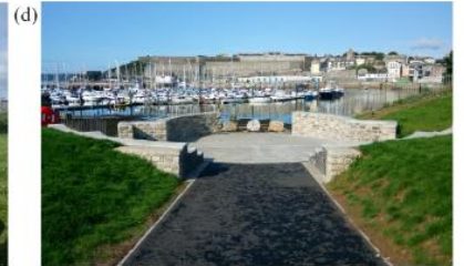
Photographs showing the lower slip road and the Intervention (open-air theatre) at T2
