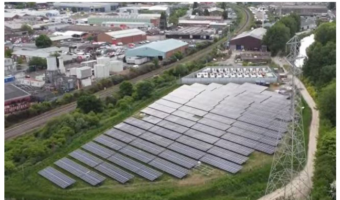
The Water Lane solar farm.
