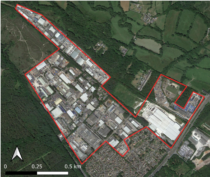
The Heathfield Industrial Estate lies between Newton Abbot and Bovey Tracy close to the A38 Devon expressway, it is home to about 200 businesses.
