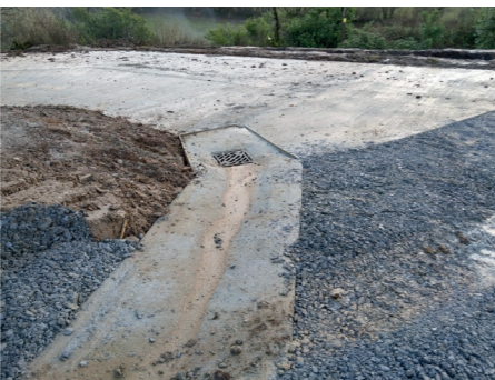
Figure 5 Cross drain and resurfaced track in the Barnstaple and Yeo catchment.
