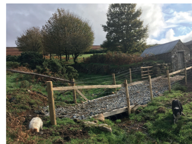
Figure 10 Re-siting of access to field and watercourse fencing installed to prevent livestock access; photo by Devon Wildlife Trust.
