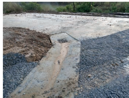
Figure 5 Cross drain and resurfaced track in the Barnstaple and Yeo catchment.
